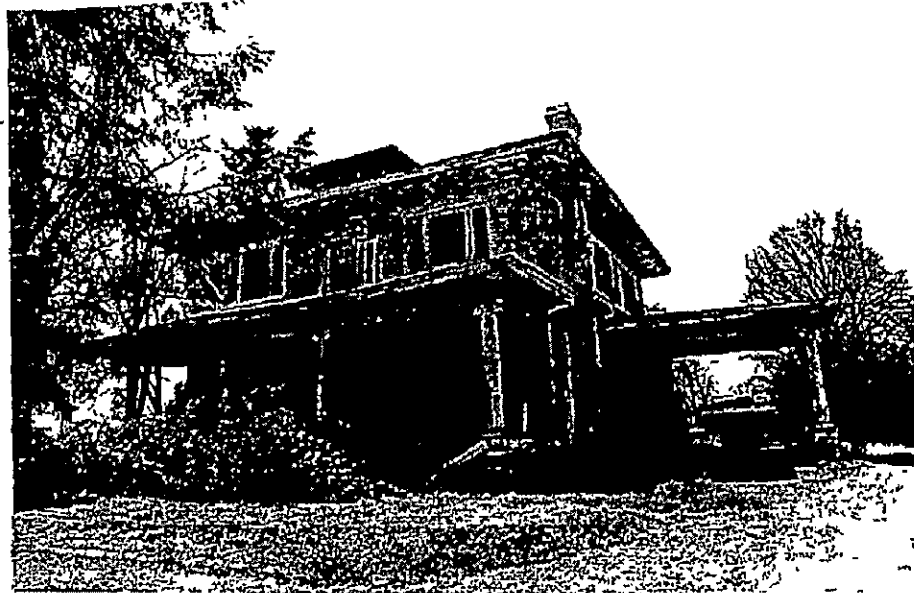
Figure 20 CK-524, Bonfield House
