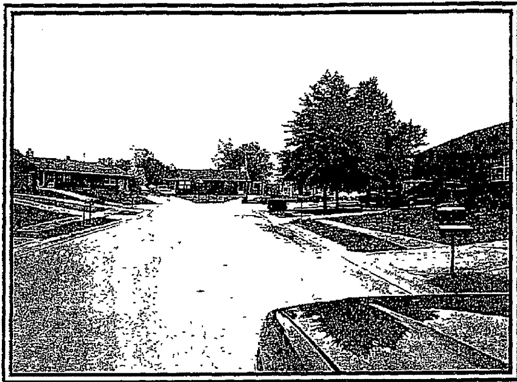
Figure 7. Photograph of the study corridor from Country Club Drive, facing east.
